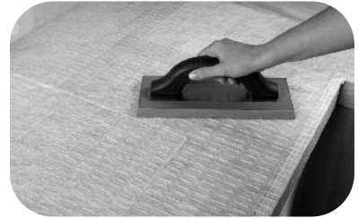
Flatten air bubbles and creases.
